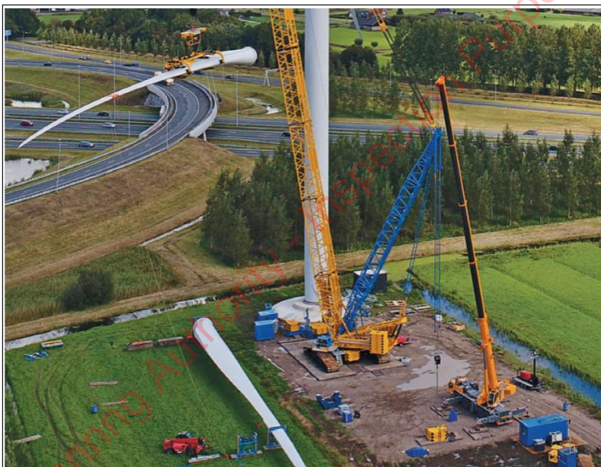
Figure 5-7: Typical finished Hardstand on a Wind Farm (Source: www.windfarmbop.com )
