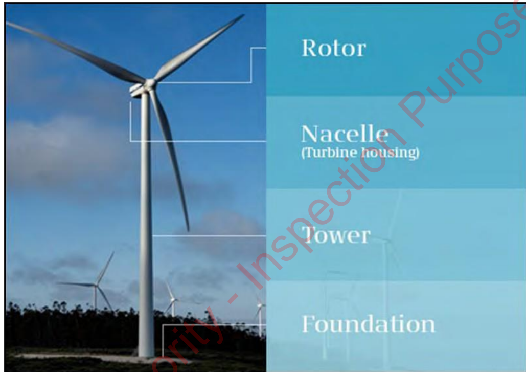
Figure 5-5: Typical Wind Turbine Components
